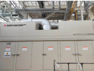
Cogeneration system deployed at the Itoham Yonekyu Foods' Nishinomiya Plant
